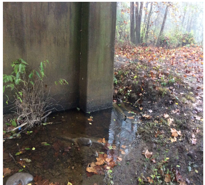
PHOTO 2 Description Looking back at bent 3: local scour at column 1.
