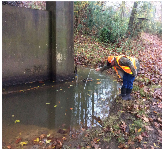
PHOTO 1 Description Looking back at Bent 2: a scour hole near column 2. (28" deep where measurement was taken)
